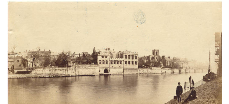
View of the Guildhall before its late 19th and early 20th century extensions. Note the prominence of the former Friary river wall and St Martin Le Grand. The west bank is shown prior to the creation of the riverside walk and a boat is loading/unloading coal by the warehouse (©York City Council - Imagine York).
