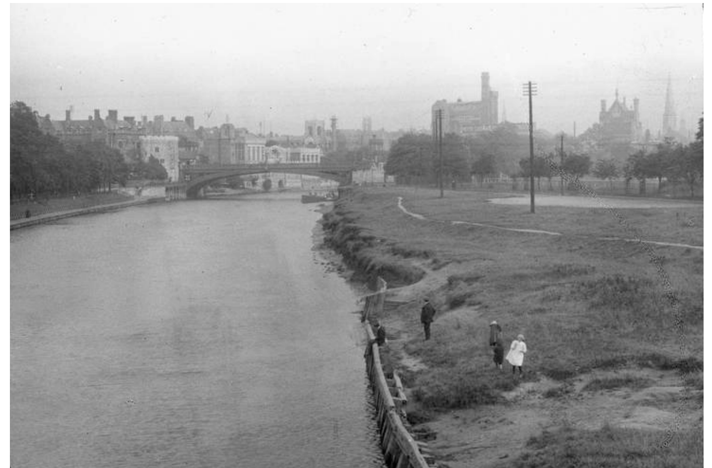
The view from 1912 illustrates the formerly more open unplanned aspect of the west bank of the River Ouse. Without the formal public walk and flood defences, this was a managed flood plain. In the background from left to right are: the waterworks tower, the Guildhall, St Martin Le Grand, Rowntree Cocoa works, Walker's Horse Repository and the spire of All Saints Church on North Street (©York City Council - Imagine York).
